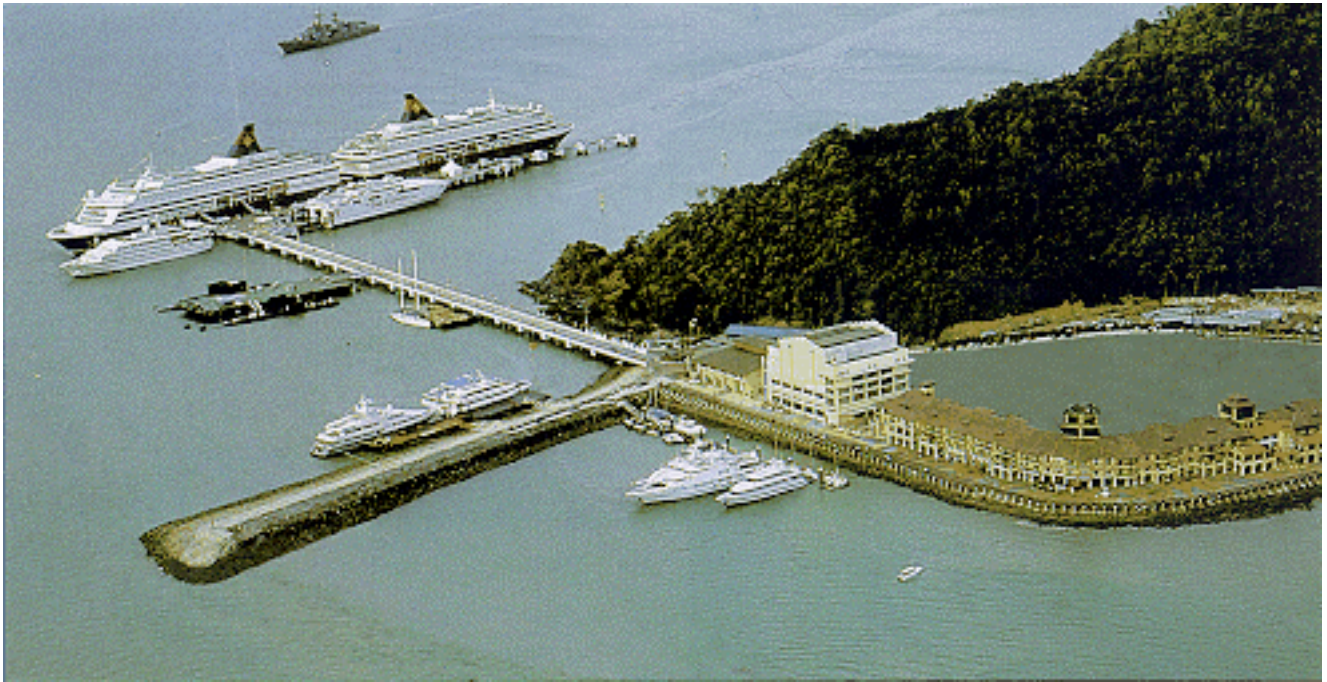
Star Cruises jetty located beside Awana Porto Malai, Langkawi
