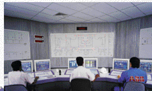
Central control room at the Kuala Langat Power Station
