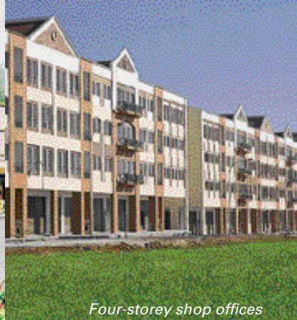
Four-storey shop offices
