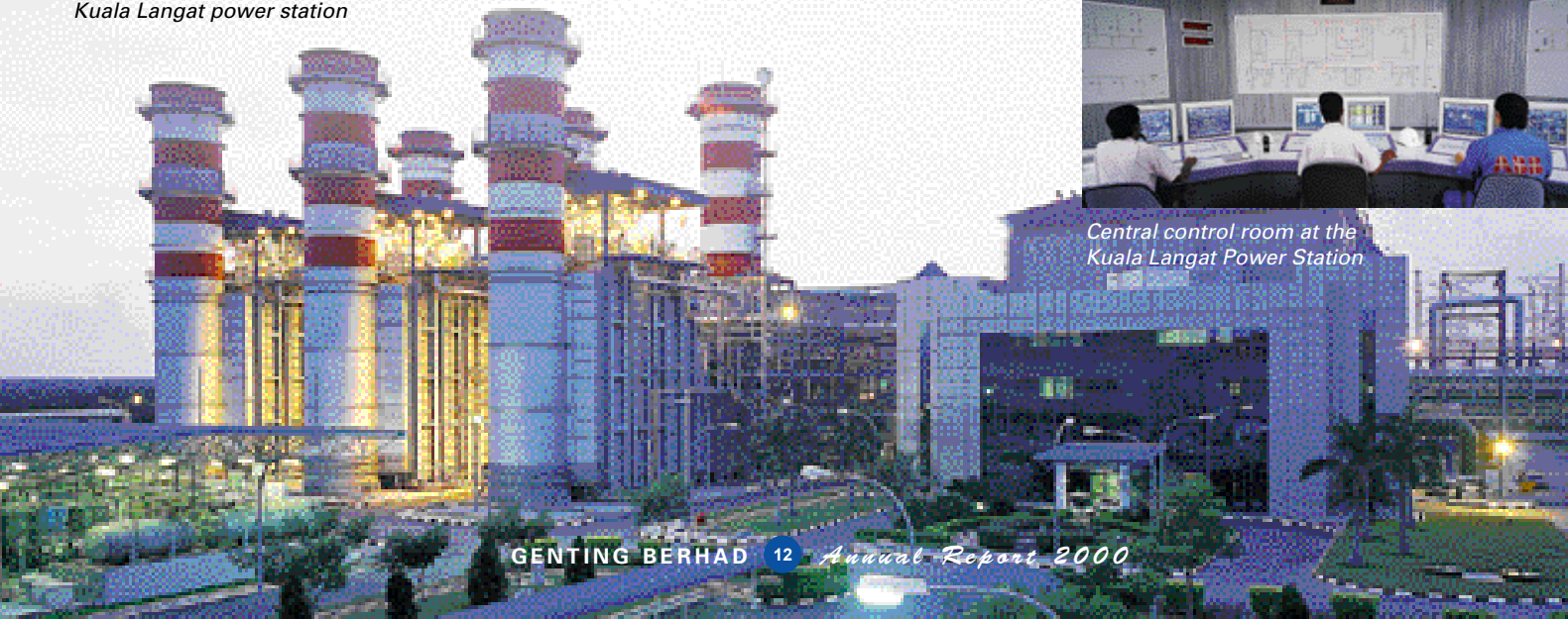
Heat recovery steam generators at Kuala Langat power station
