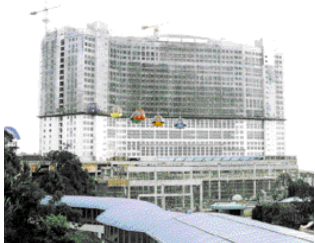
The first phase of First World Hotel under construction
