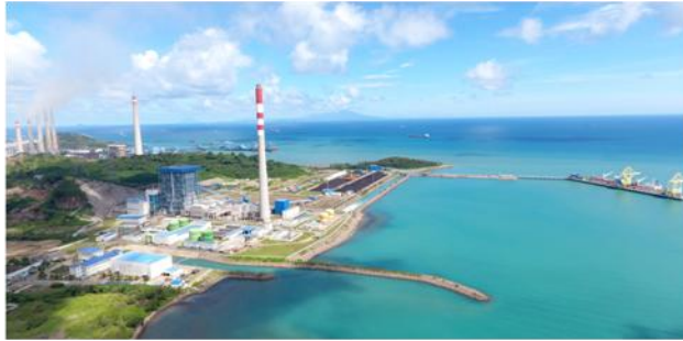
Indonesia – Banten power plant
