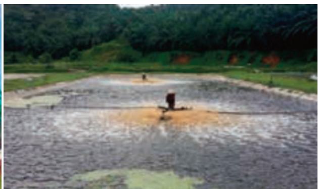
Mixers and aerators installed in effluent ponds
