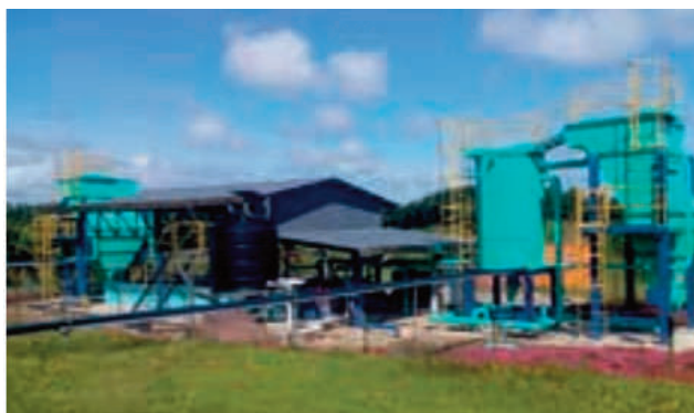
Bioflow and membrane bioreactor plant at Genting Mewah Oil Mill
