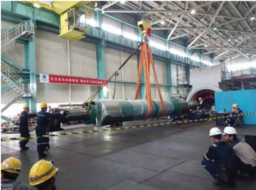
Banten power plant's scheduled major outage - Insertion of Generator Rotor and inspection of Generator Stator
