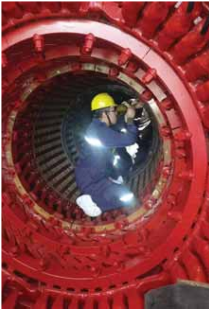
Banten power plant's scheduled major outage - Insertion of Generator Rotor and inspection of Generator Stator
