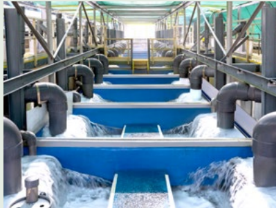
View from atop our foam fractionators cleaning and filtering seawater used for S.E.A. Aquarium
