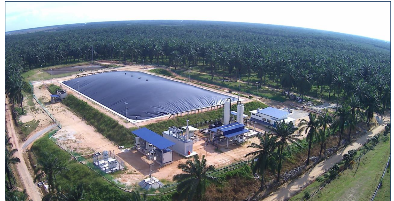
GENTING AYER ITEM OIL MILL Biogas-Capture Facility, Johor, Malaysia
